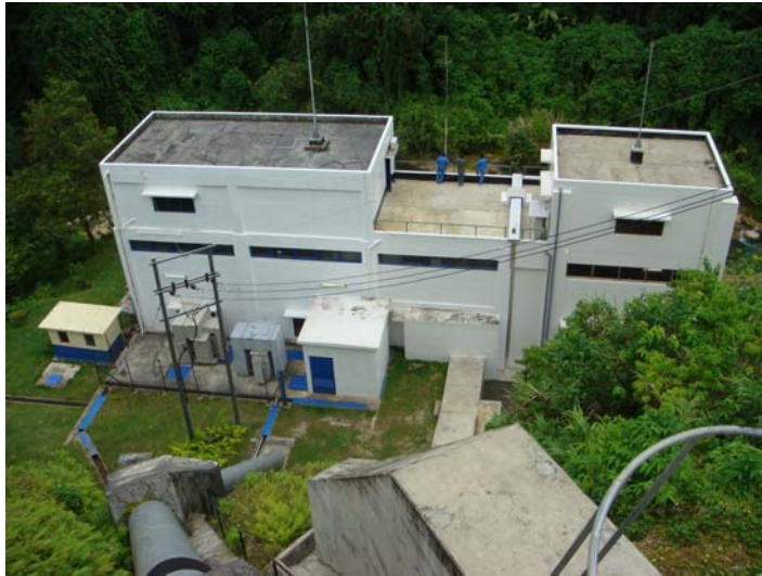
Sarakata Hydro Plant, Santo (source: IPA)
